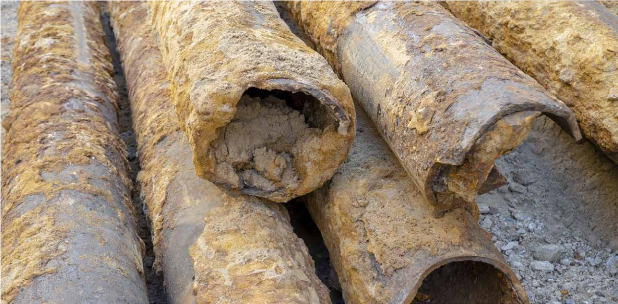
Corroded steel pipes
